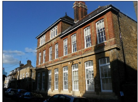
Former Thanet School of Art & Crafts (Department of Building), New Street, Margate
